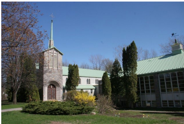
PHOTO New Metal Roof on the CPUC Sanctuary and Fellowship Hall.
