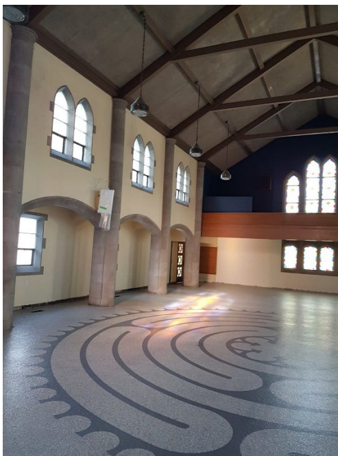
PHOTO: New Polished Concrete and coated floor with labyrinth
